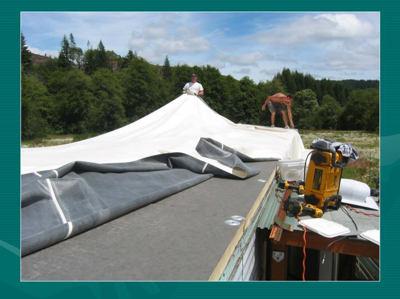
Singlewide Manufactured Home Receives a New Roof Under the New EPDM Roof is a 4" Solid Core Styrofoam Insulation
